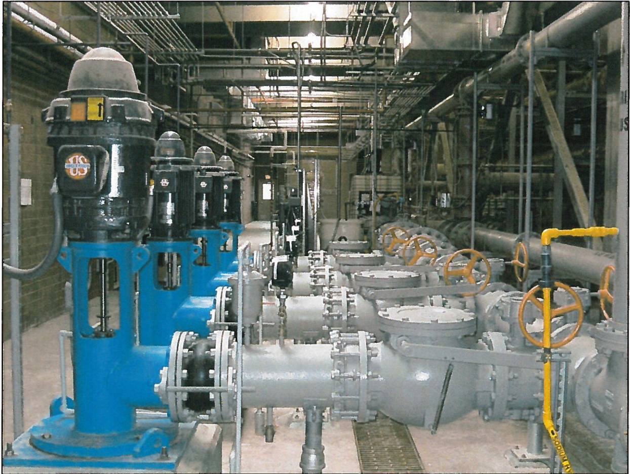
Above are the tertiary effluent pumps at the Lone Tree Creek Water Reuse Facility (LTCWRF).
