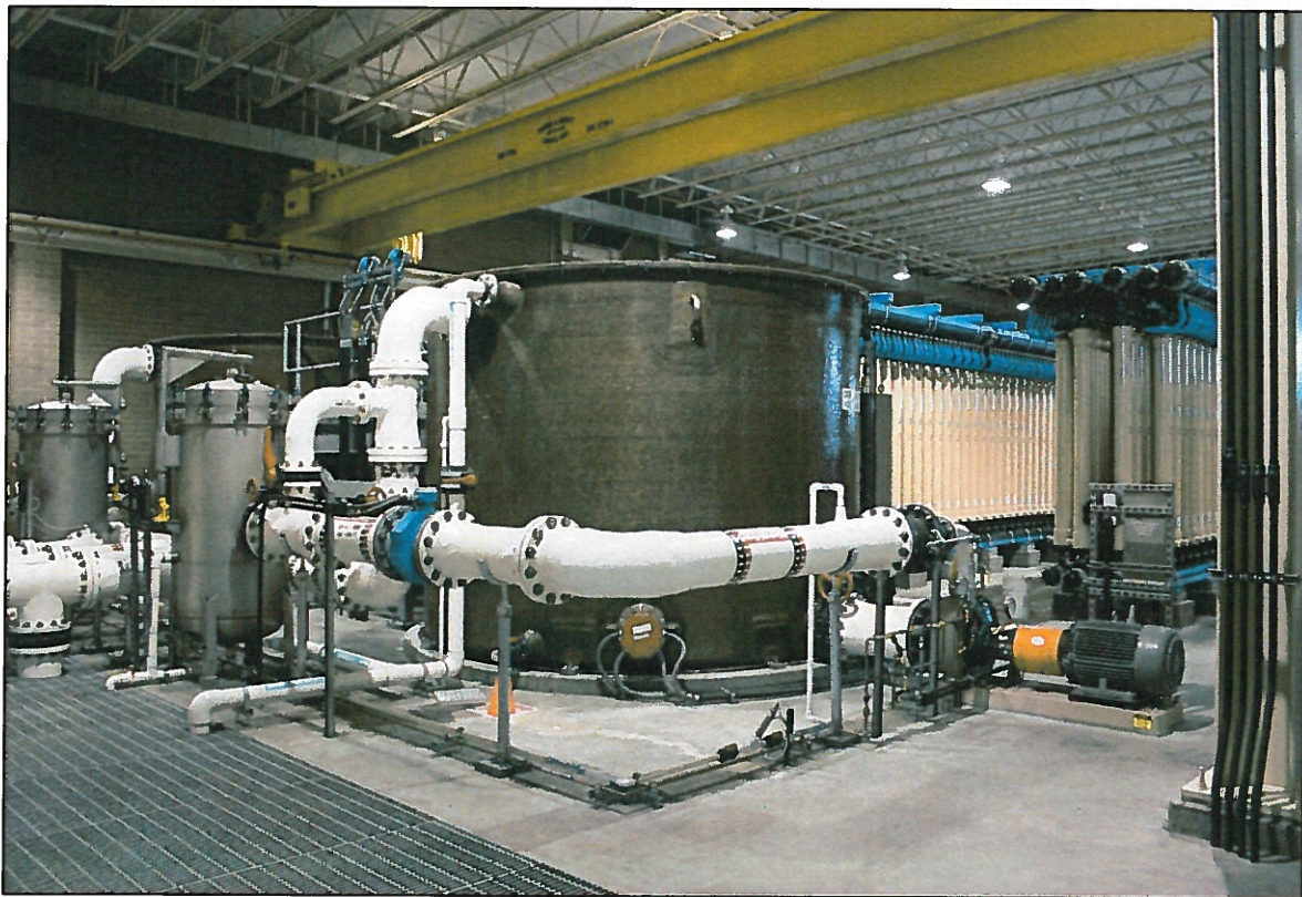
Pictured above is the Clean in Place system at the Joint Water Purification Plant (JWPP); to the right is the Pall Microfiltration System currently in use to filter potable water.
