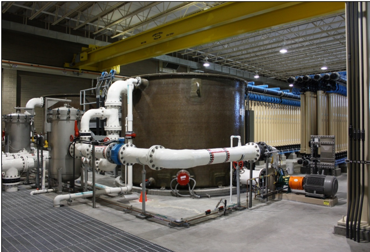
Pictured above is the Clean in Place system at the Joint Water Purification Plant (JWPP); to the right is the Pall Microfiltration System currently in use to filter potable water.
