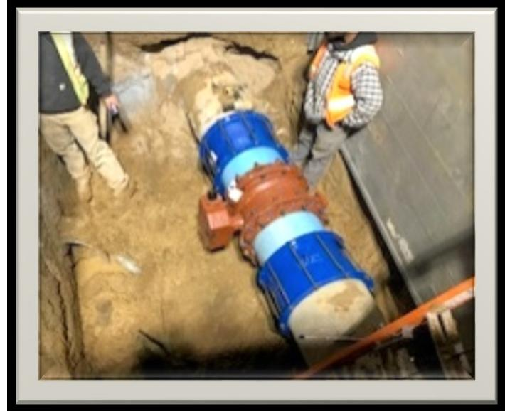
The valve identified with the highest risk of failure was replaced on November 6, 2021, located at the southwest corner of Arapahoe Road and Revere Parkway. This valve has been in service for more than 40 years, and is crucial in maintaining potable water service to customers west of Revere Parkway on Arapahoe Road. This 18" valve wouldn't isolate, which would have caused major issues if there was a water main break to the west.
