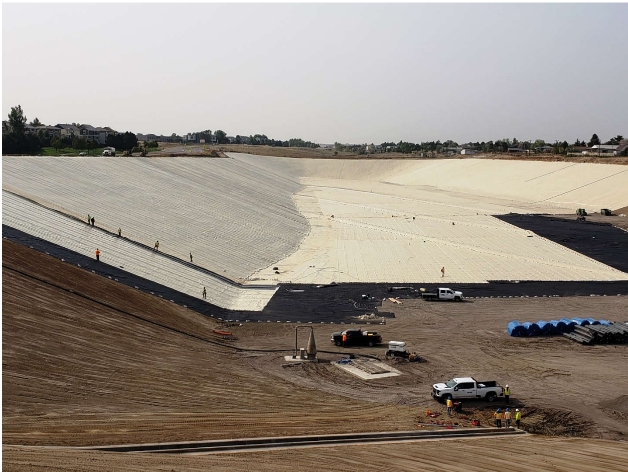
Above is the installation of the Chamber's Liner in 2021
