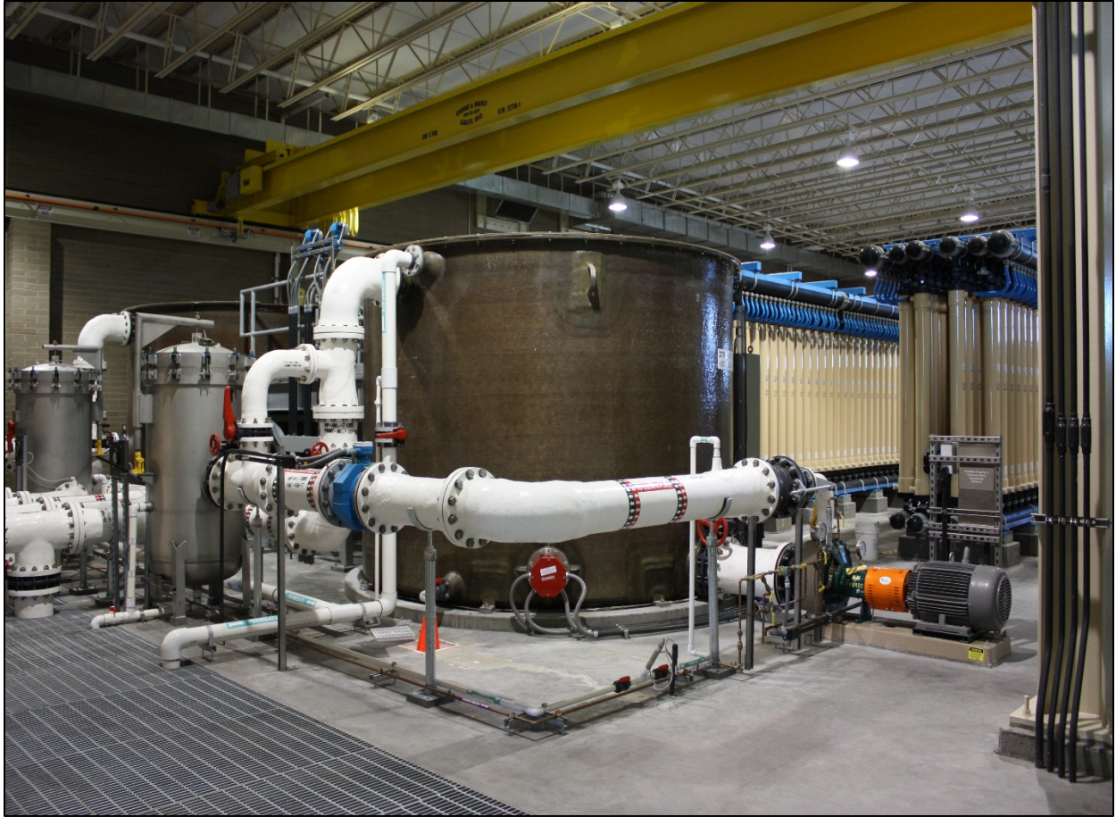
Pictured above is the Clean in Place system at the Joint Water Purification Plant (JWPP); to the right is the Pall Microfiltration System currently in use to filter potable water.
