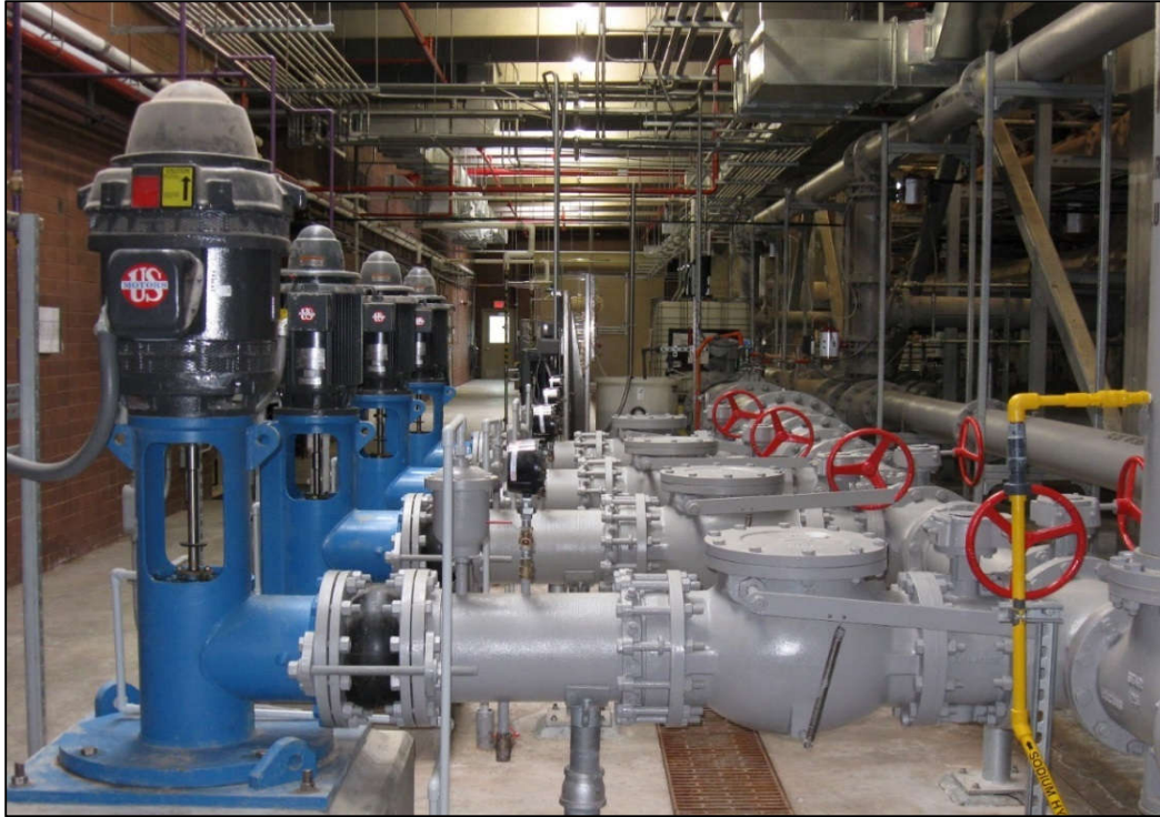
Above are the tertiary effluent pumps at the Lone Tree Creek Water Reuse Facility (LTCWRF).
